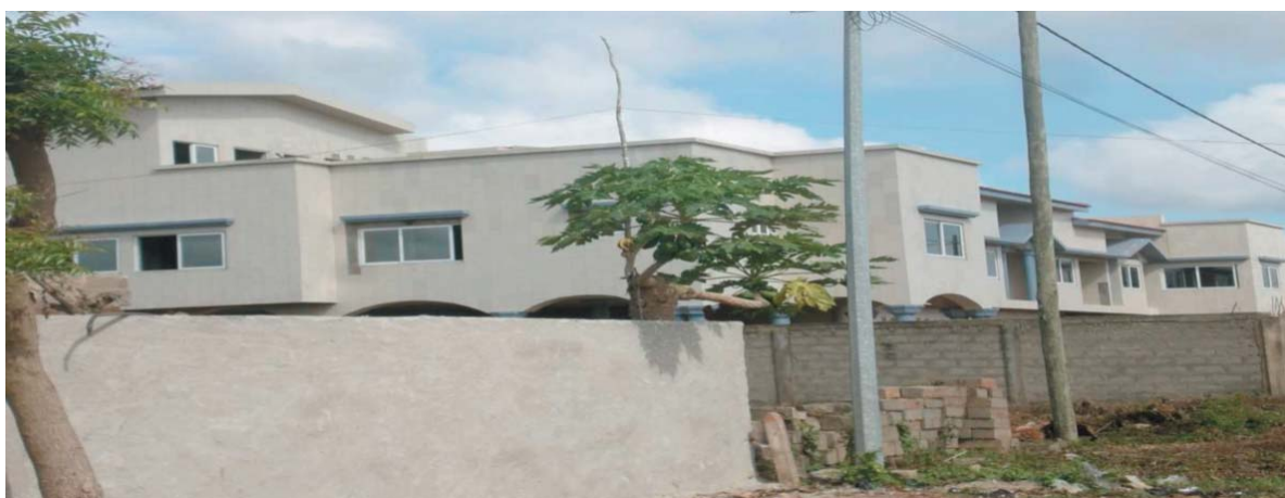
Figure 2: A completed unit at Arcon Ville (Picture taken by Bernard Tayoh)
