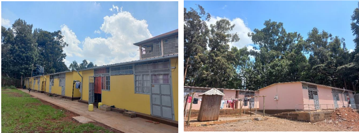
Fig 1: The Kwangu Kwako Limited (KKL) projects in Kawangware comprise of 17m 2 studios renting for Kshs 9,000-10,000 (USD 67-75) per month. The projects are owned by two small landlords and KKL does the construction using precast concrete panels and fabricated metal components. Kawangware is a unique settlement within Nairobi, in that residents hold title to their land. The area includes a mix of single and multi-storey walk-ups as well as less formal settlements.
