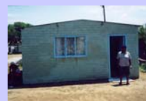
Subsidised core house
