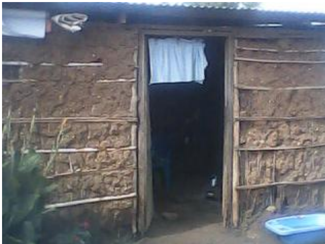
Fig. 2: An example of a Tukul/gottya (built with mud and sticks)
